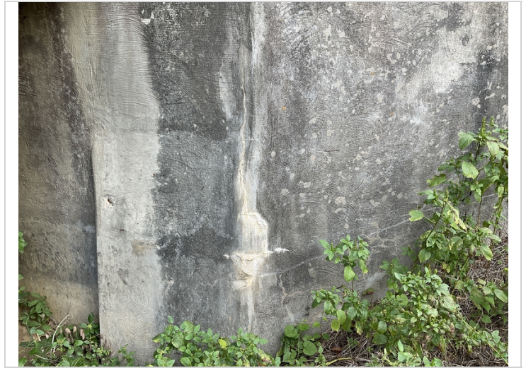
Abutment 2 efflorescence
