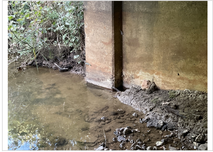
Bent 2 column 1 abrasion
