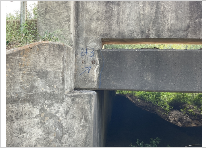
LT side @ Bt 3 efflorescence
