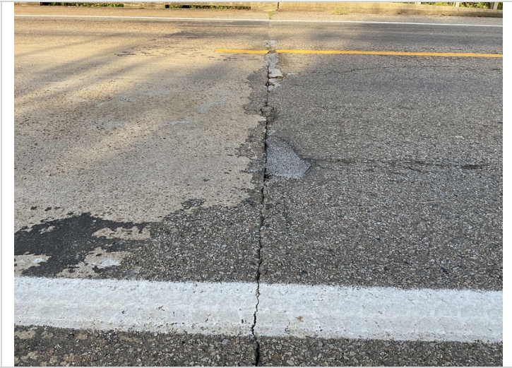
Asphalt overlay impacting joints
