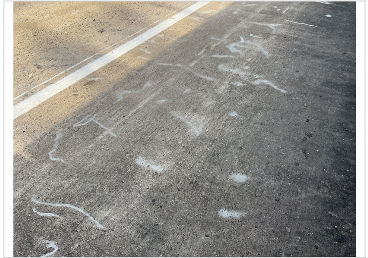
Deck cracking sealed in the past
