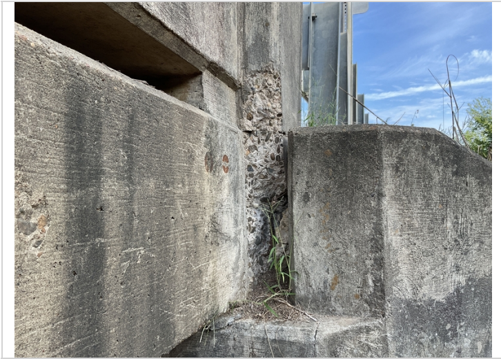
End of bridge Rt side spall with rebar exposed
