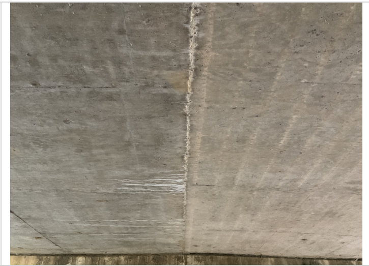
Efflorescence on underside of slab
