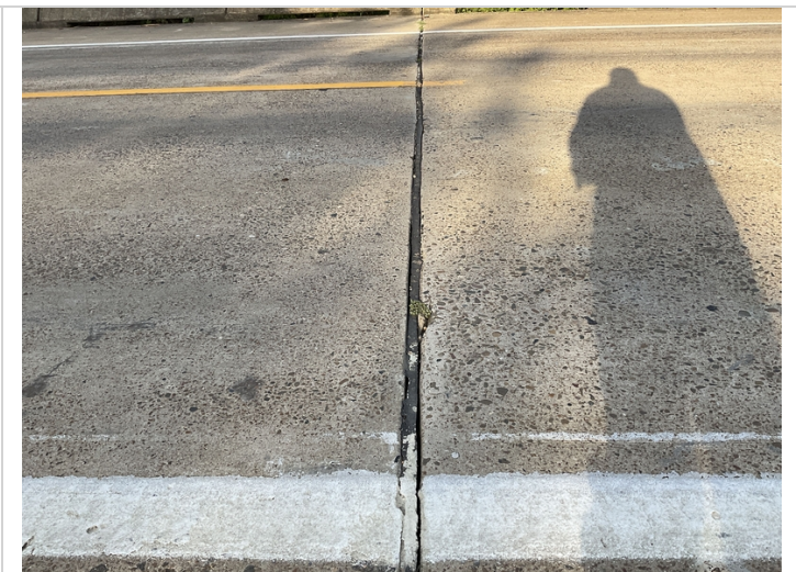
Leakage to pourable joint seal
