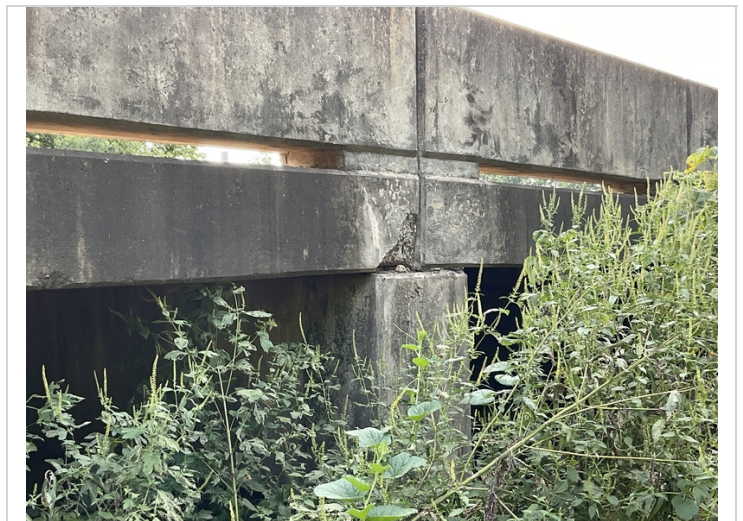
Spall with efflorescence cracking @ LT side bent 2
