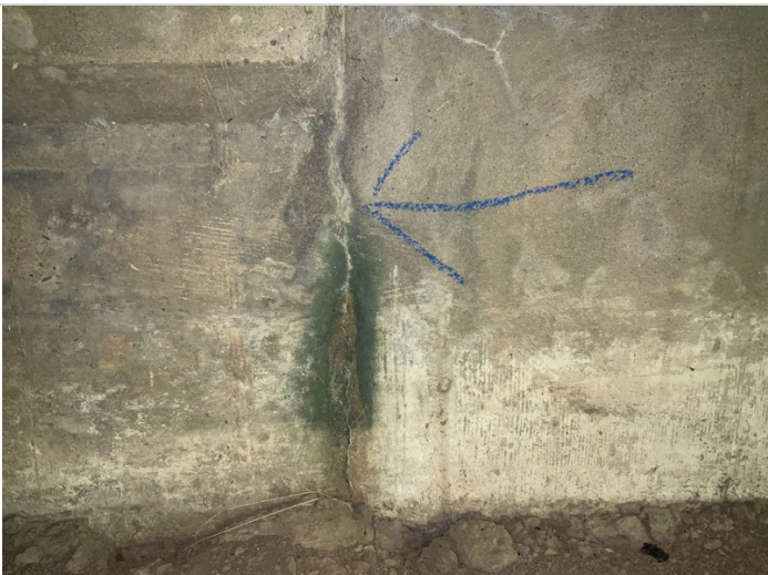
Abutment 1 cracking
