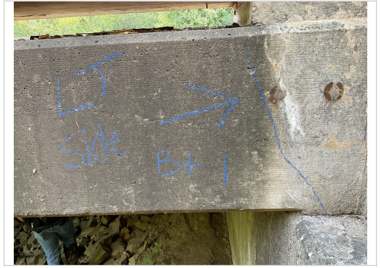
LT side @ Bt 1 efflorescence
