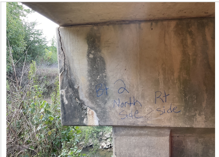
Bt 2 Rt side Delam with efflorescence
